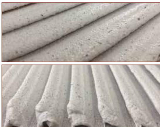
**STESURA COLLA CON SPATOLA DENTI INCLINATI**
